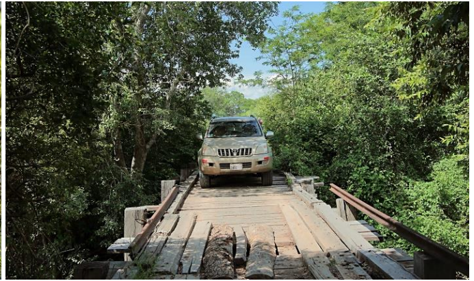
Fig. 57: Bridge across Rio Tucabaca.
